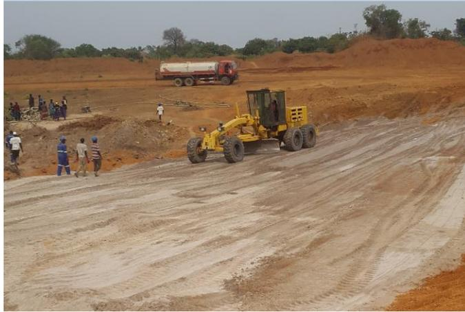
**Spreading of filter blanket Down Stream of the Dam Embankment**
