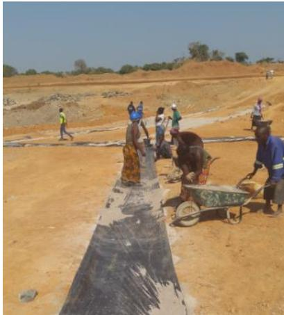
**Excavation, Filling and covering of filter drains on down stream side**
